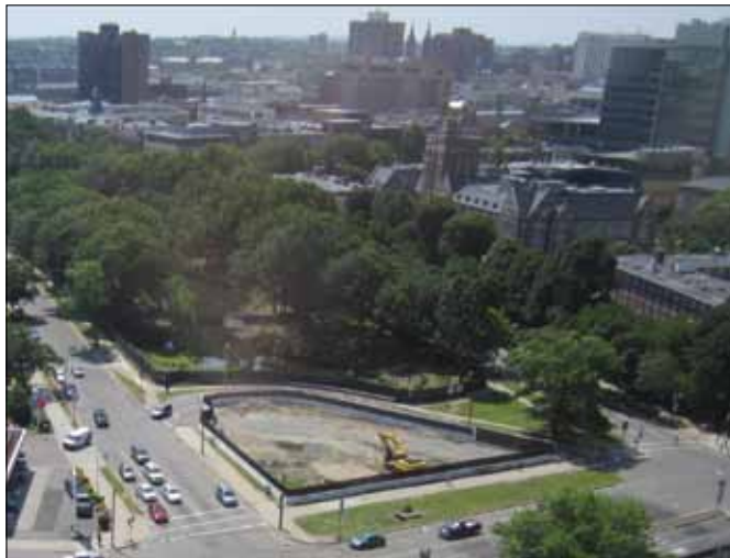
View of Upper Fens Pond before construction. Note jughandle road to be eliminated.
