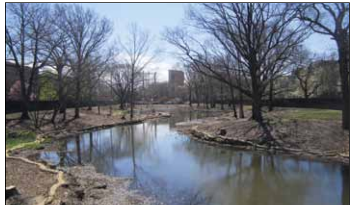
Upper Fens Pond in April 2013 after clearing for Phase 1 construction.
