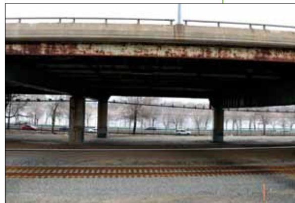
Current condition of the turnpike viaduct
