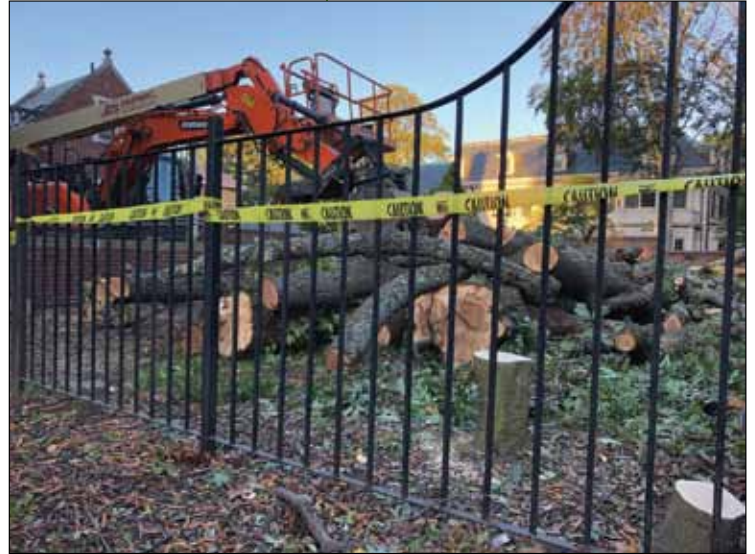
An example of the preconstruction clear cutting the by-law will prevent.
