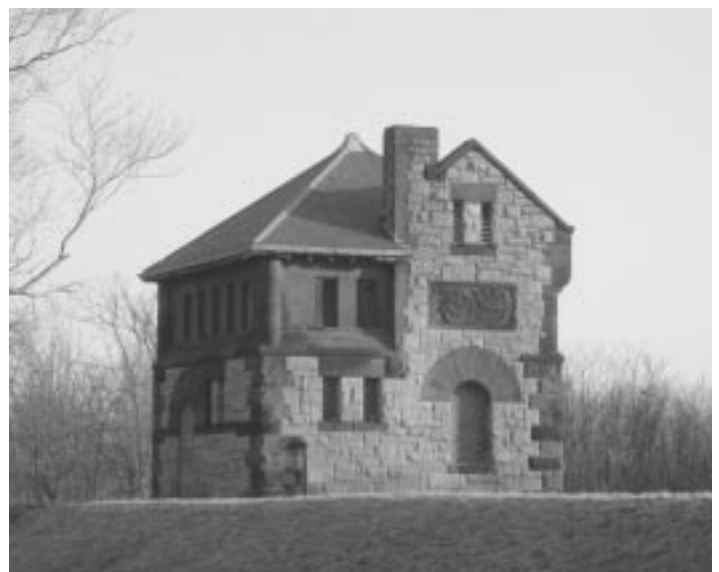
Pumping station at Fisher Hill. Photo by Marian Lazar
