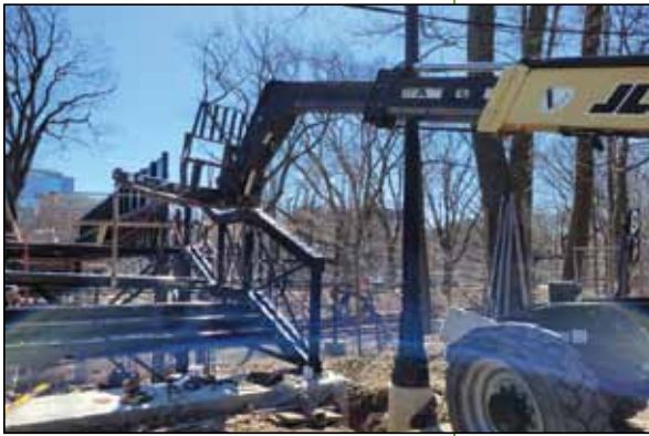
The return of the footbridge: From 5 AM to 8 AM, the entire main span was lifted over the trees and placed on the vertical steel columns
