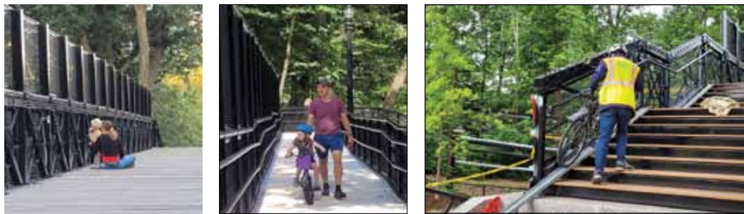
The bridge now fully accessible and a wonderful place to view the trains.
