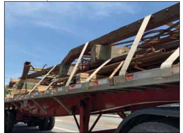
Above: First step in restoration: The bridge is disassembled and loaded on a truck for restoration at the Aetna facility in Rhode Island.
